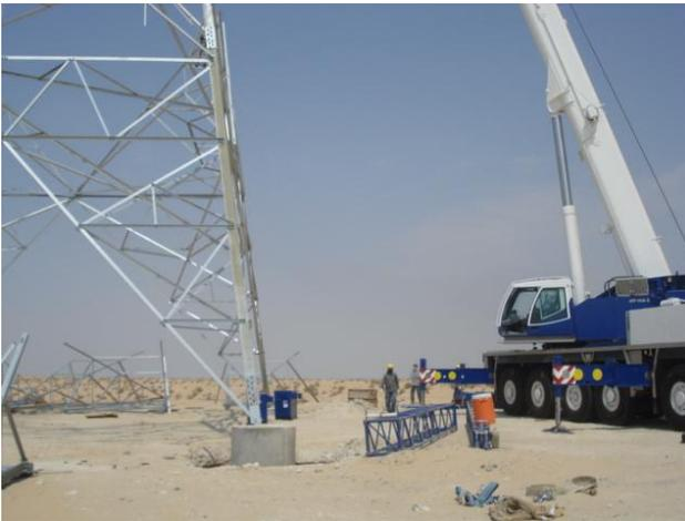
**Figure 5 - Construction of Tower near Ghunan Substation**
